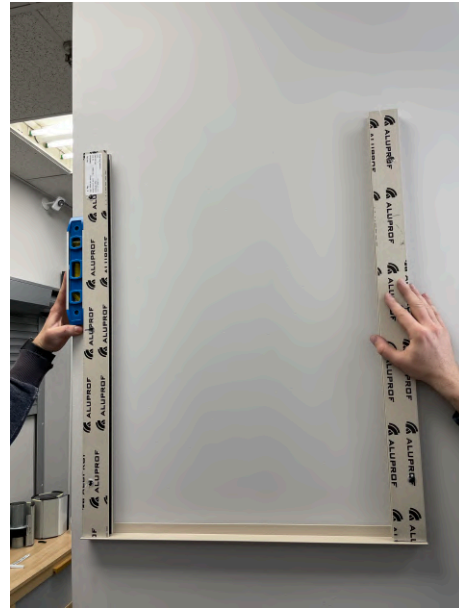
Checking level position of Guide Rails.
