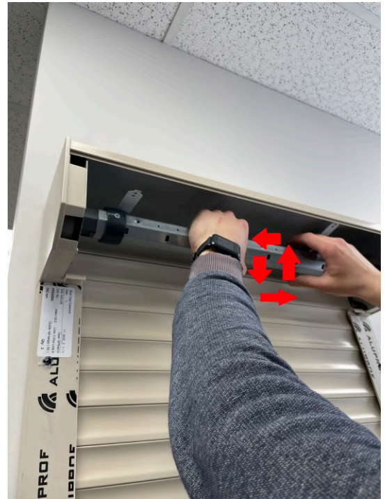
7.2 Roll all available tape to the plastic wheel using shaft
