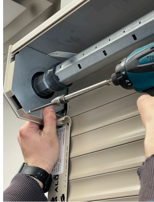
6.4 Screw the tape to the special hole in the plastic wheel
