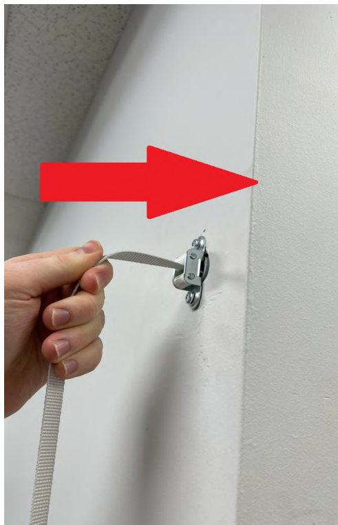
5.3 Put the tape through the tape slider, so it will stick out of the wall at another side
