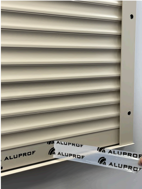
Peeling off protective plastic.
