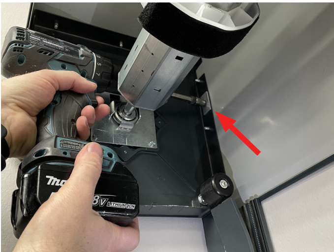
Securing left side of Box.
