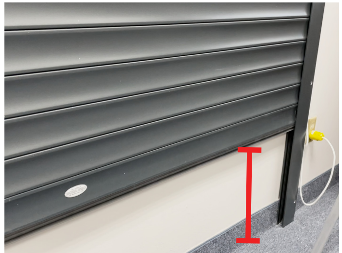
The curtain has reached its factory default bottom limit.
