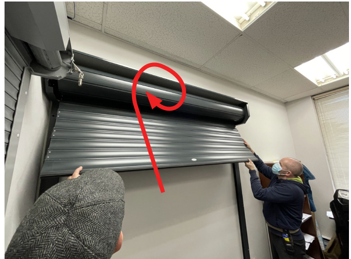
Hold Curtain when rolling Curtain into Box.
