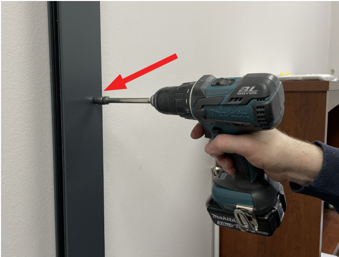
Securing Guide Rails in place.
