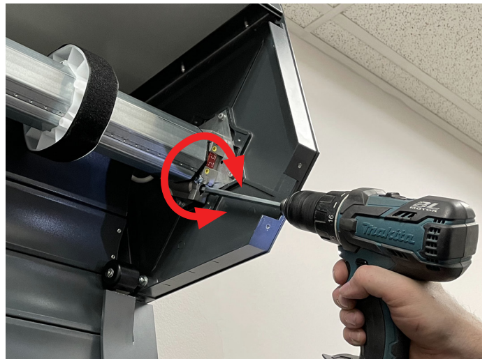
An example of tool used to operate the manual override.
