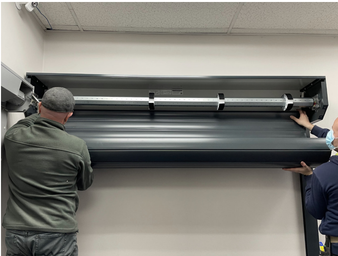
Lifting Curtain behind and over the Shaft.
