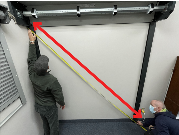
Measuring diagonal of Guide Rail position.
