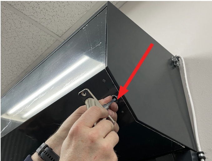
Installing Manual Override Assembly.
