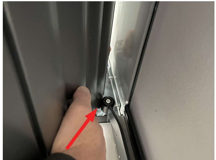
The Curtain should be above the rollers inside the Box.
