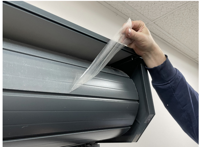
Peeling off protective plastic.
