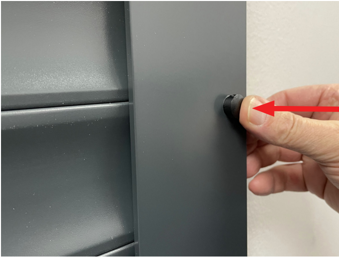
Plugging up mounting hole.
