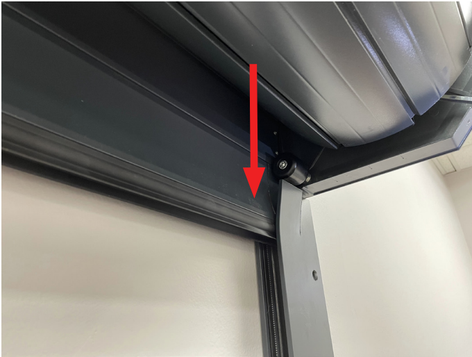
Curtain positioned to feed into Guide Rails.
