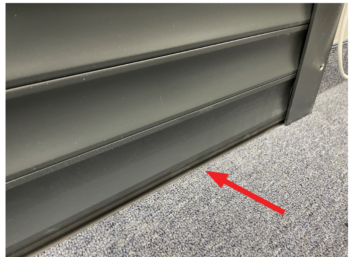
Adjust lower limit till the Curtain is firmly at the bottom.
