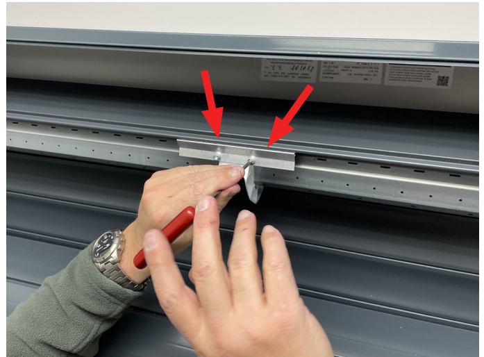
Secure the Hangers to the Shaft Collars.
