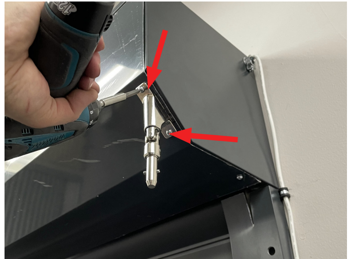
Securing Manual Override Assembly in place.
