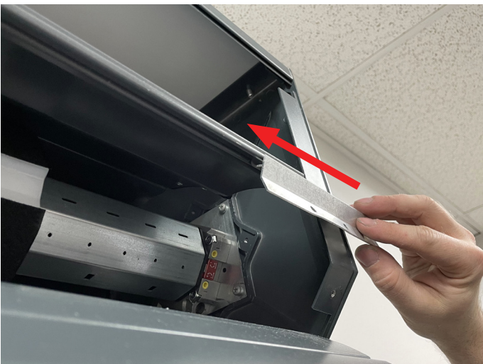
Slide Hangers onto the end of the Curtain.
