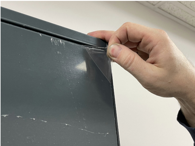
Peeling away protective plastic from Box Cover.
