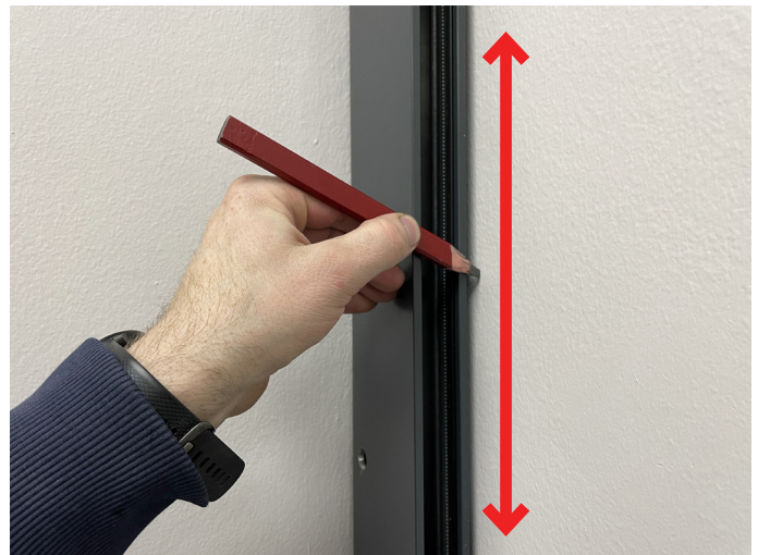
Marking Guide Rails position.
