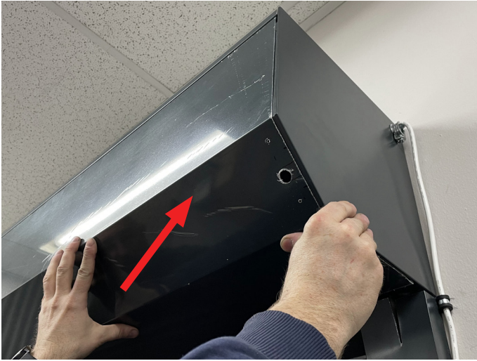
Mounting Box Cover in place.
