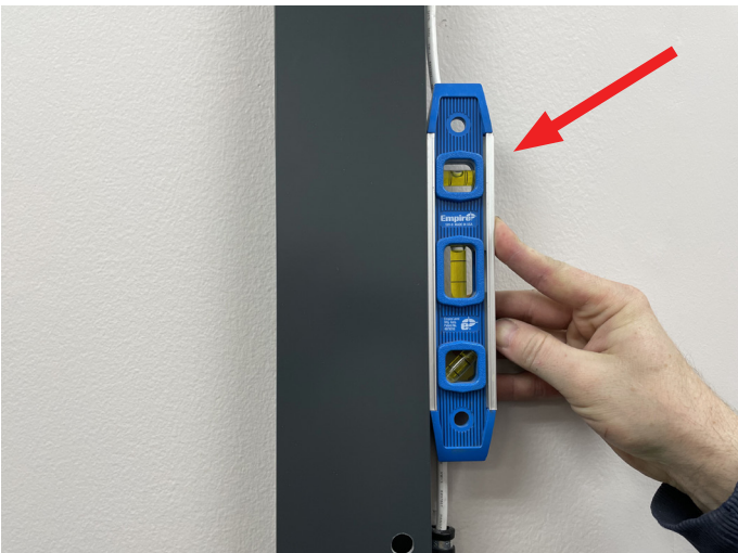
Checking level position of Guide Rails.
