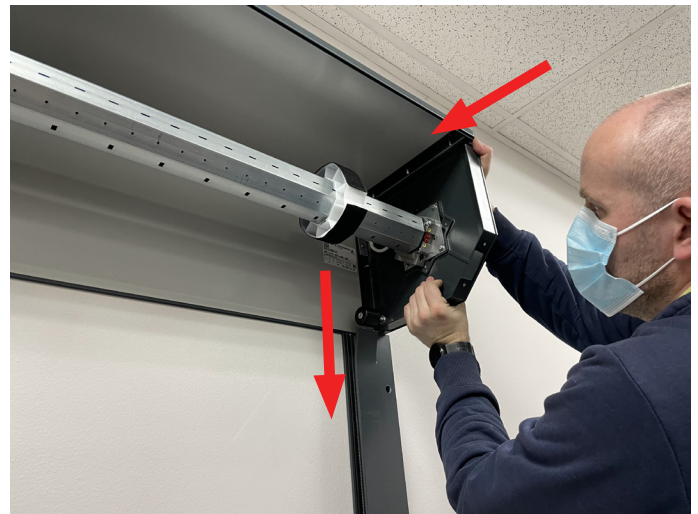
Placing Box in position.
