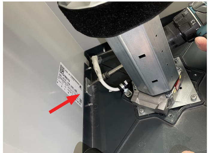
Securing right side of Box.
