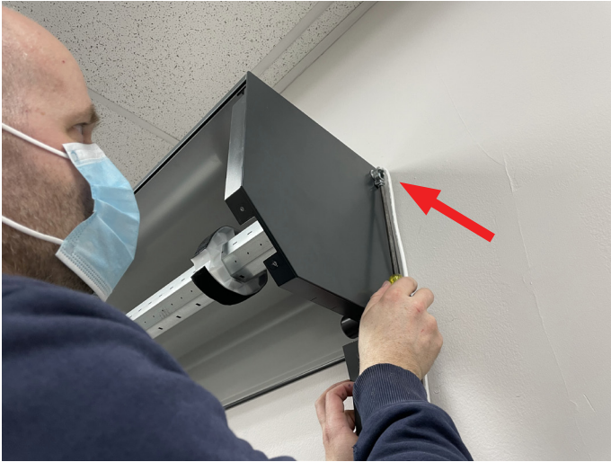
Securing power cable.
